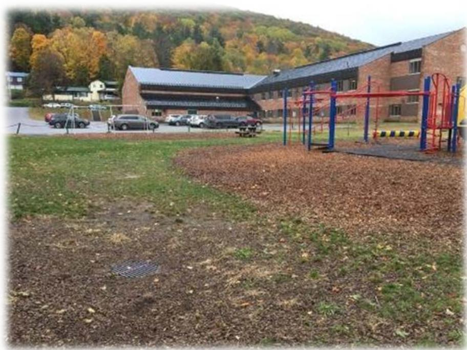
**Figure 4: School 001 (northern) site. The inlet to the existing dry well is shown in the foreground. The system of chambers would be installed underground directly off the edge of the parking lot’s paved area.**
